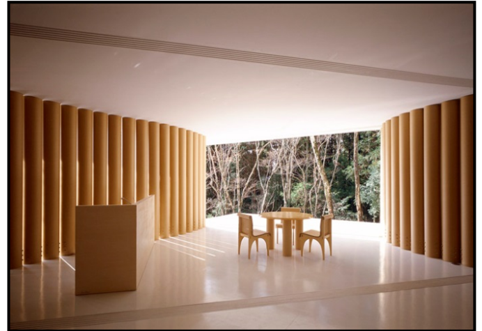
FIGURE 8b: Shigeru Ban, inside view of Paper House , Lake Yamanaka, recycled paper tubes, wood and glass, Japan, 1994–1995.
