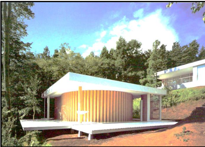
FIGURE 8a: Shigeru Ban, Paper House , Lake Yamanaka, recycled paper tubes, wood and glass, Japan, 1994–1995.
